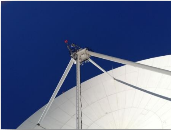
X-band Feed is located at the prime focus
